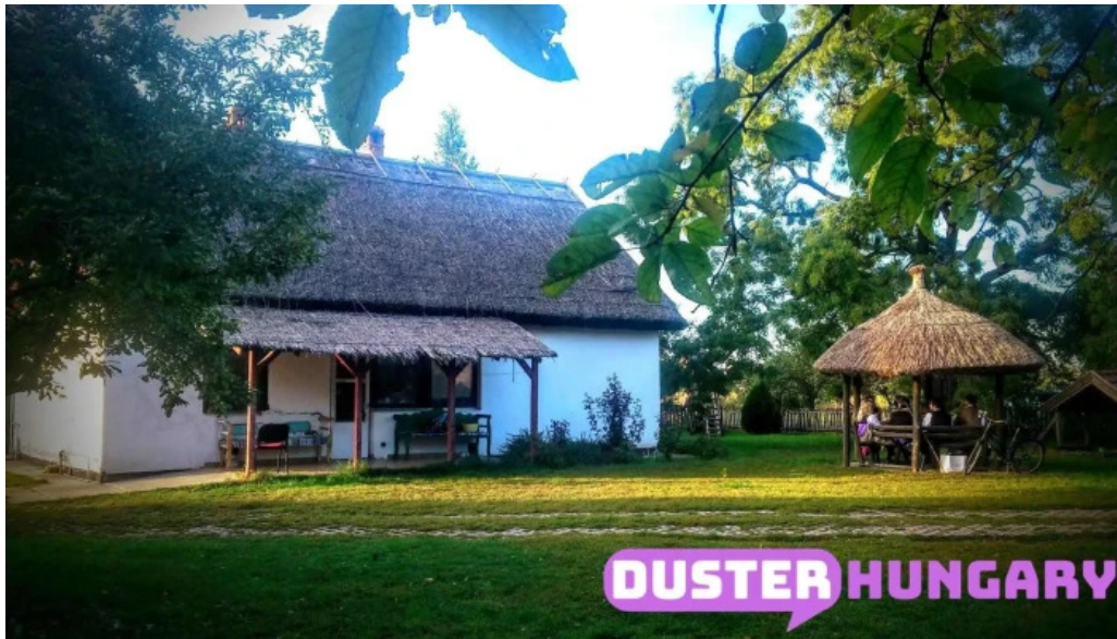
Koroknai porta barand kulso
