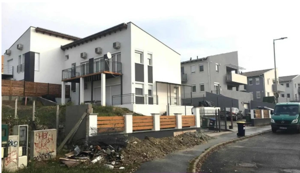
Vmr technic kft kulso
