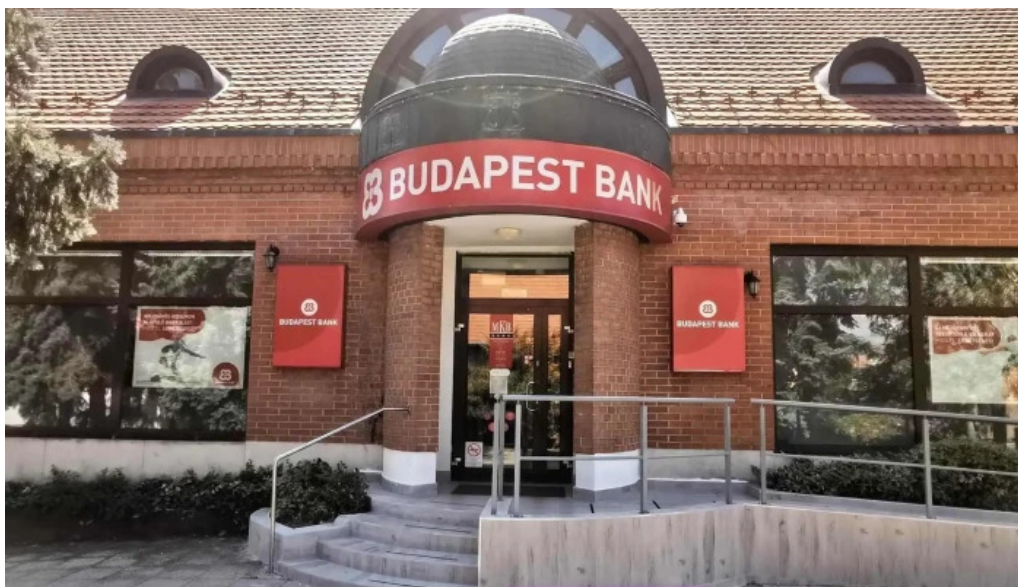
Mbh bank rackevei fiok kulso
